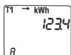
Energy counter: Set tariff: 1 (T1) dir.: imp. (→) Value: 123.4 kWh Currently: active (A)
